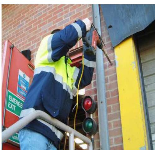
If locating the SCP outside, find a suitable route for the cable through the building wall, and drill cable hole as shown.
